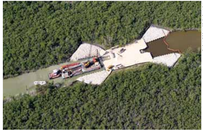
Figure 3. Aerial view of nearly completed dam at East Cape Canal, Cape Sable, Everglades National Park. The dams are expected to add resilience to upstream freshwater ecosystems by reducing unnatural intrusion of saltwater into the area.
